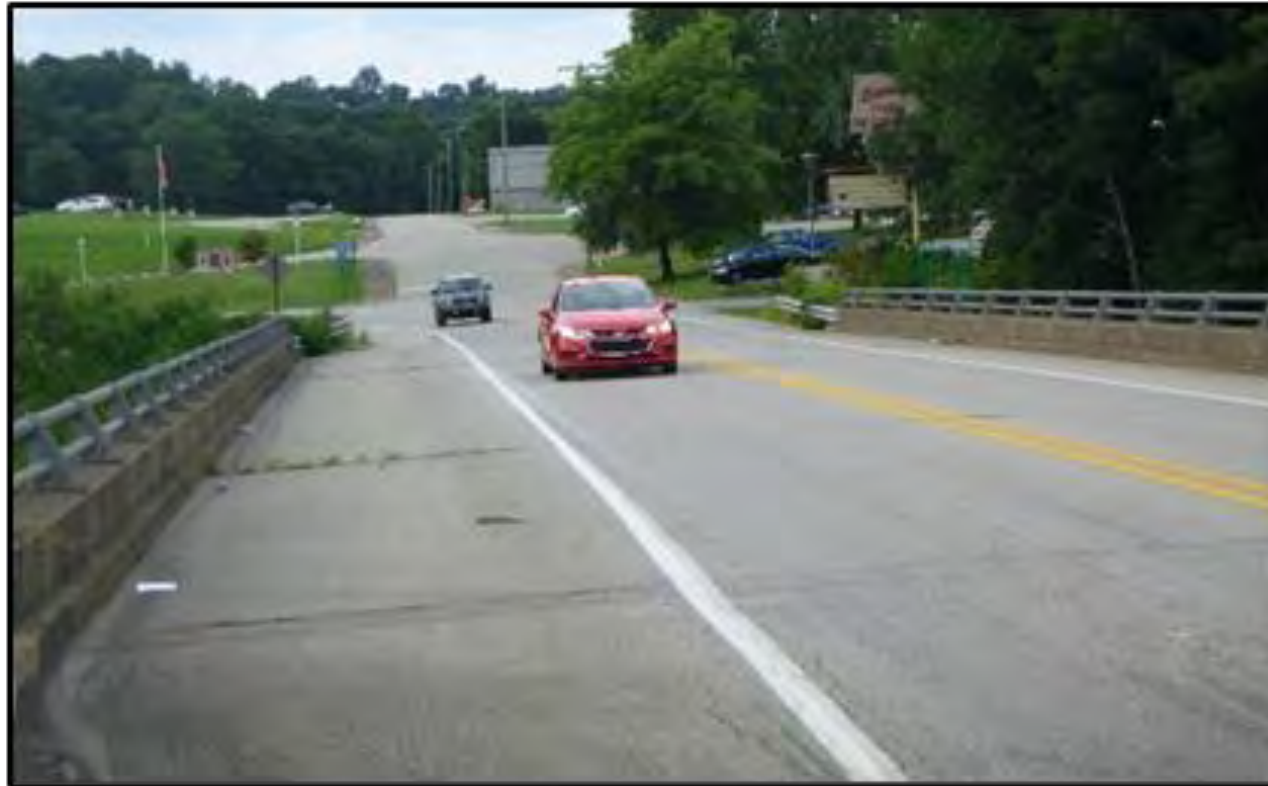
SR 2027 (Maple Drive) Looking Northbound
