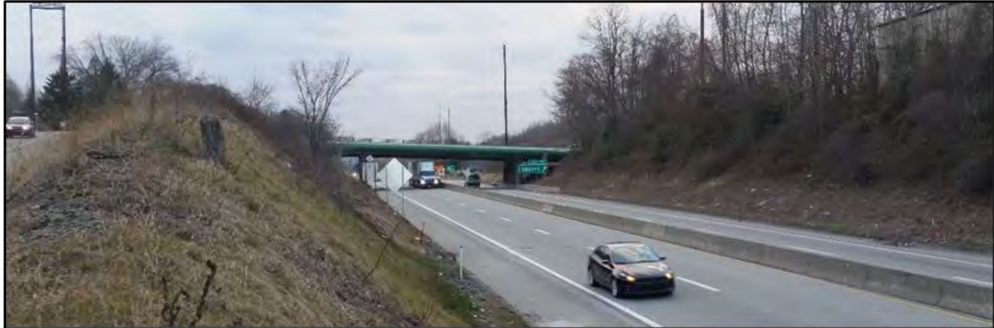
SR 2027 D10 Bridge Looking West along I-70
